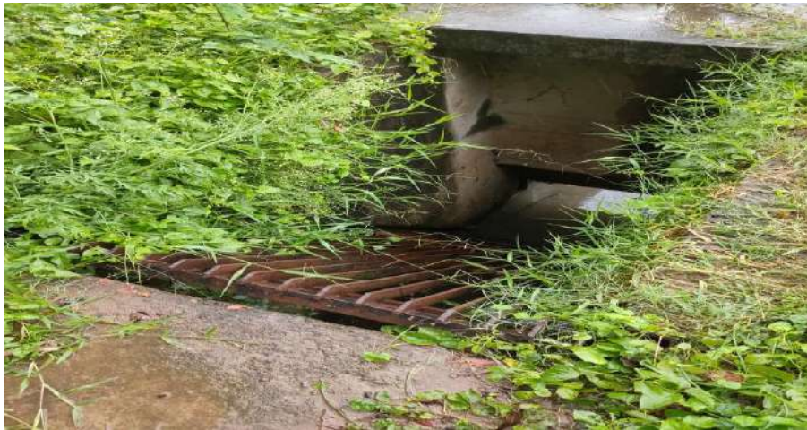
33 MLD STP at Mattagajpur Cuttack
