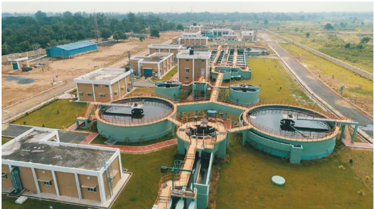
16 MLD STP at Mattagajpur Cuttack
